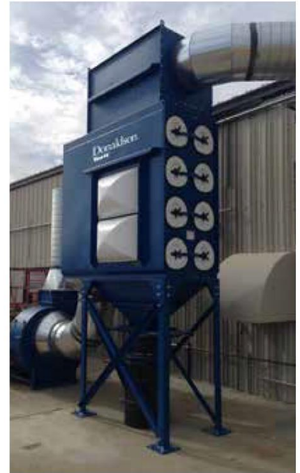
DFO on Plastics Routing 16,000 cfm (27,184 m 3 /h)
