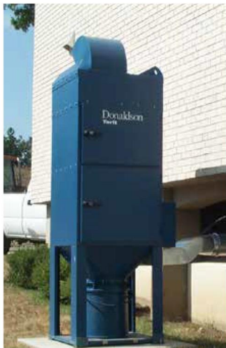
UMA - School Wood Shop 2,000 cfm (3,397 m 3 /h)
